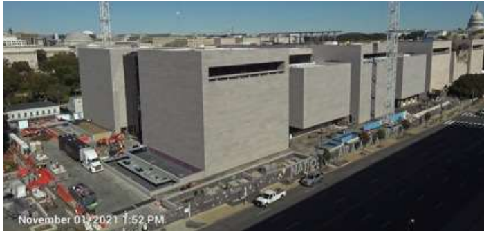
Nov 2021: Looking Northeast – Terrace/Planter Work On-going
