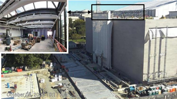
Oct 2020: Looking Northeast – Zone 1 Stone Install Complete and Install of New Topping Slab at West Terrace On-going (lower right in picture)
